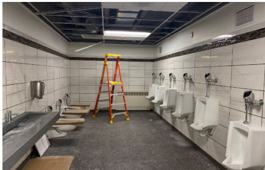
GP North Restroom Renovations
