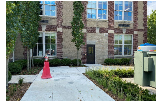
Richard ES New Secured Vestibule
