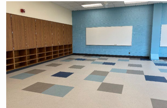
Richard ES New Ceilings, Lighting, Flooring, Millwork
